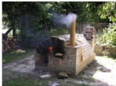
Fig. 2. Replica of a two-chambered calcination kiln in Detoul v Orlických horách during the heating before the calcination.
